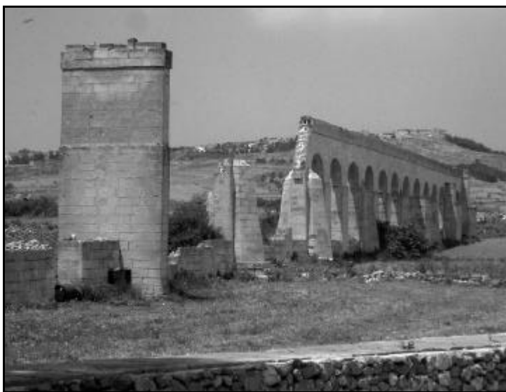
Part of the Roman aqueduct on the island of Gozo
